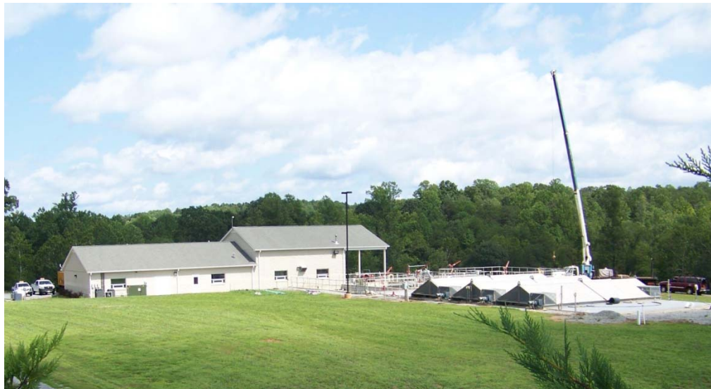
Moneta Wastewater Treatment Plant Moneta, VA
